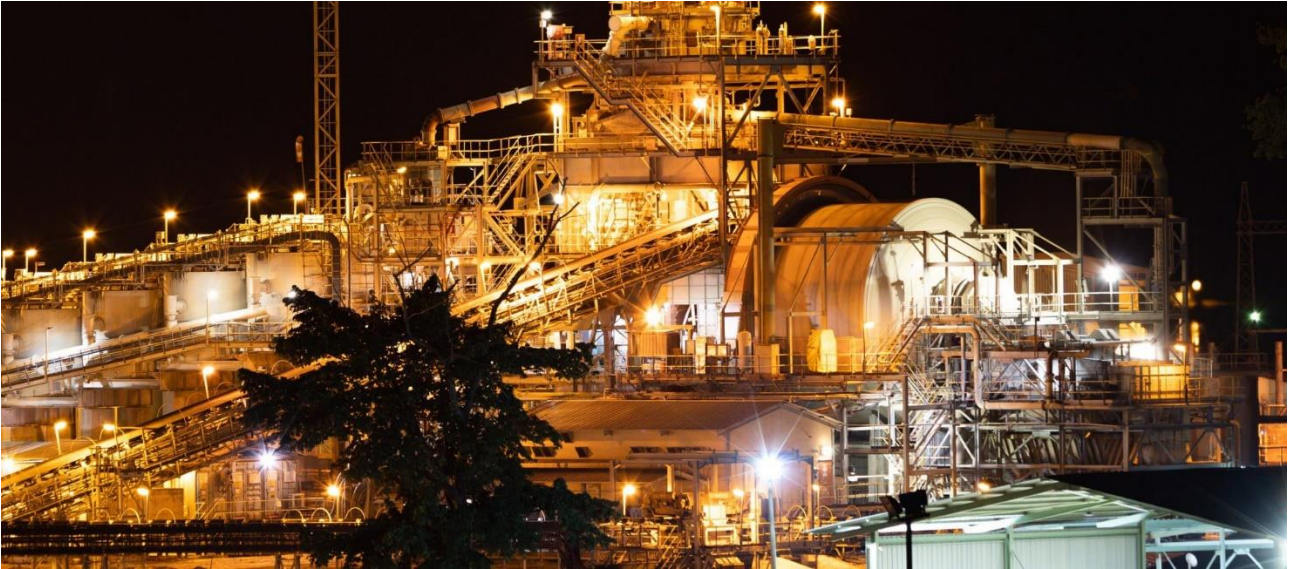
Figure 2 - The Edikan SS SAG Mill
